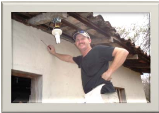
Chris Niedergeses Installing a Porch Light
